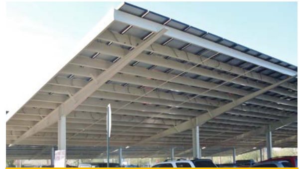
Double Cantilever- Dual Purlin - Tapered Beam
