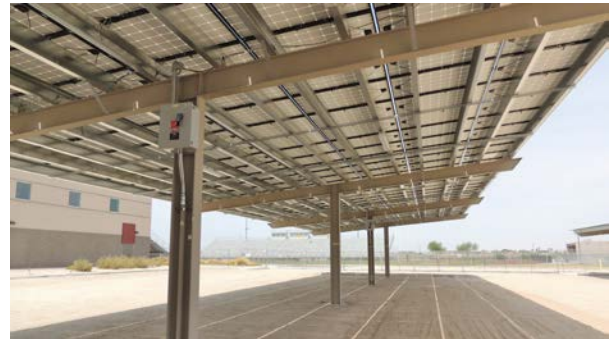
Double Cantilever- Dual Purlin - Straight Beam
