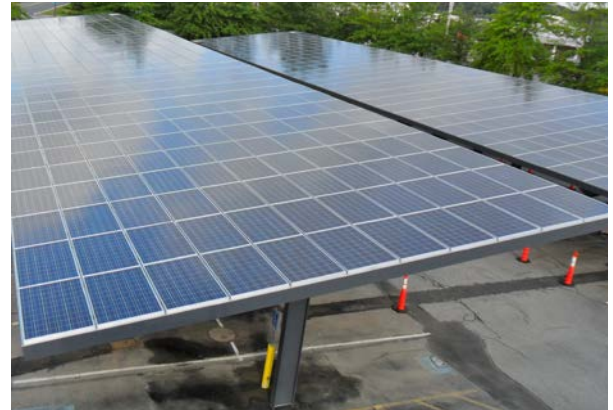
Double Cantilever- Shared Purlin – Modules
