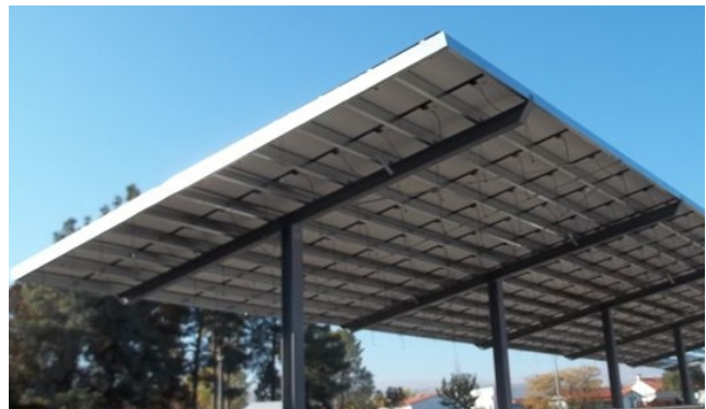
Double Cantilever-Shared Purlin-Straight Beam
