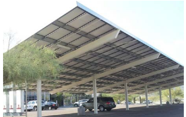
Double Cantilever- Shared Purlin - Straight Beam
