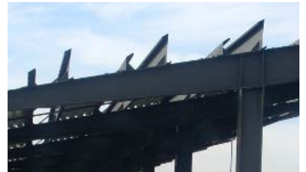
Dual Zee Purlins – Create added Tilt Angle
