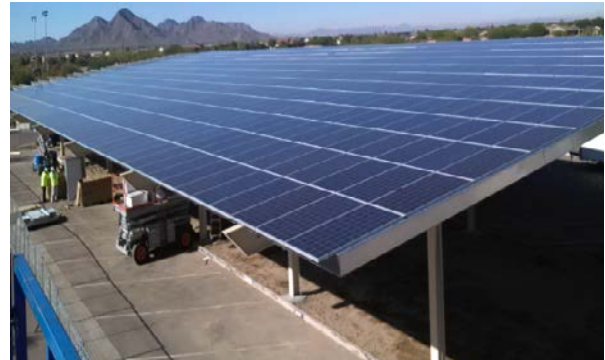
Double Cantilever – Dual Post Extends Width
