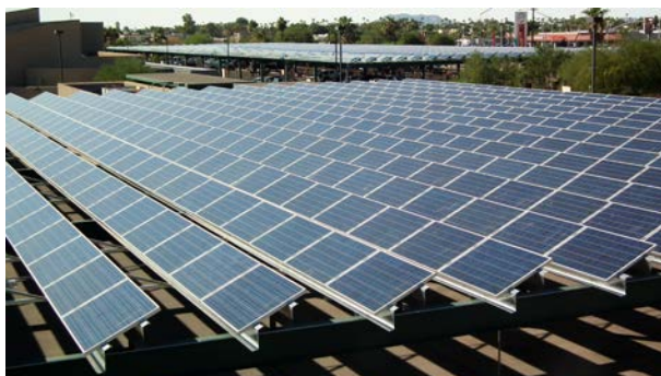
Municipal Airport Parking Lots
