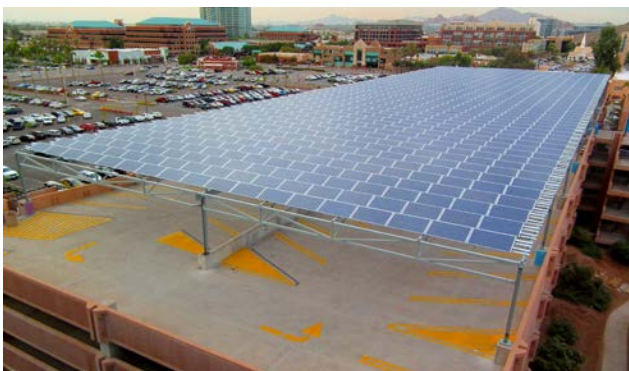
University Parking Garage Top
