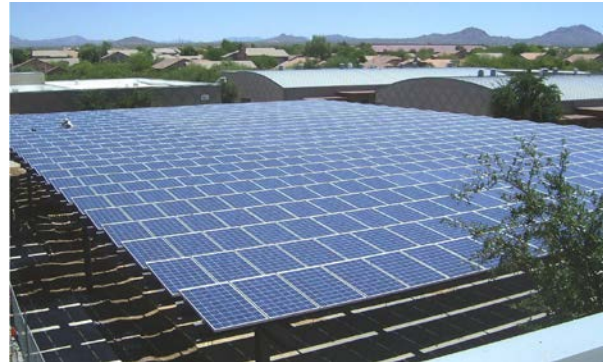
Multiple Post Canopy – School Break Area
