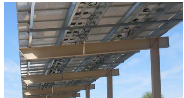
Full Cantilever- Dual Purlin - Straight Beam
