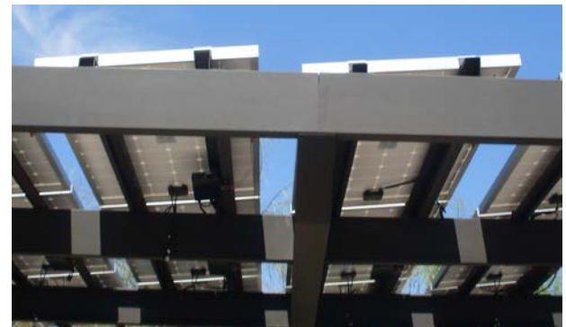
Lower Hat-Upper Z Purlin-Modules Racked 5 degrees
