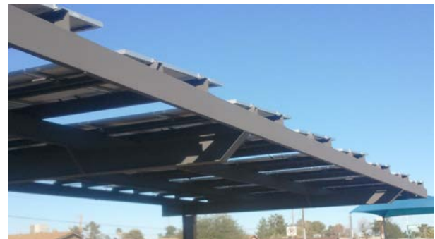
Full Cantilever- Modules Racked 5 degrees
