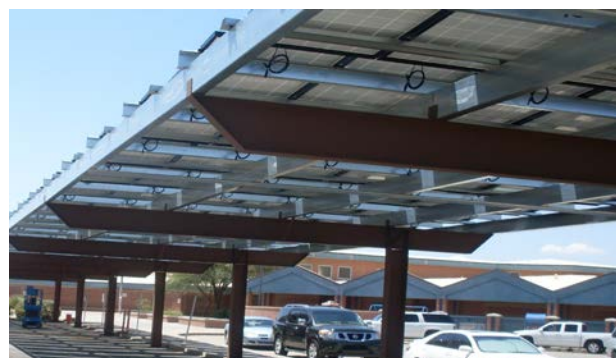
Partial Cantilever -Modules Racked 5 Degrees
