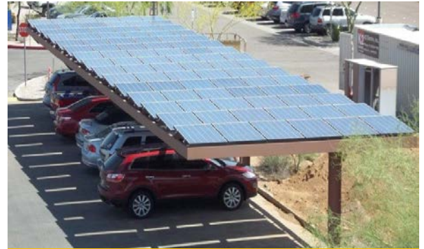
Partial Cantilever- Modules Racked 5 degrees
