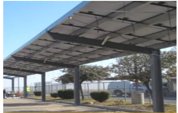
Full Cantilever - Shared Purlin - Straight Beam
