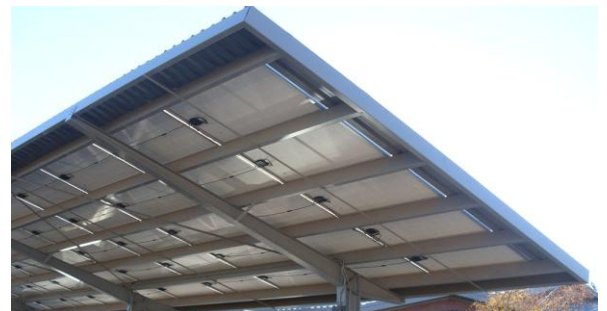
Full Cantilever- Shared Purlin - Tapered Beam
