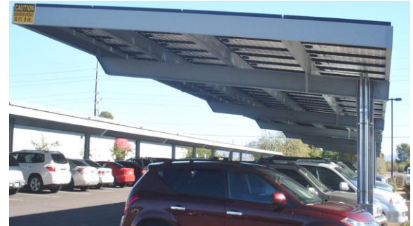
Full Cantilever - Shared Purlin - Straight Beam
