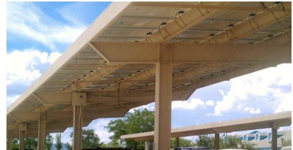
Partial Cantilever- Shared Purlin - Straight Beam
