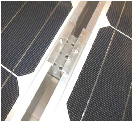
1. Position the TGMC over the support rail, snug in-between solar modules.
